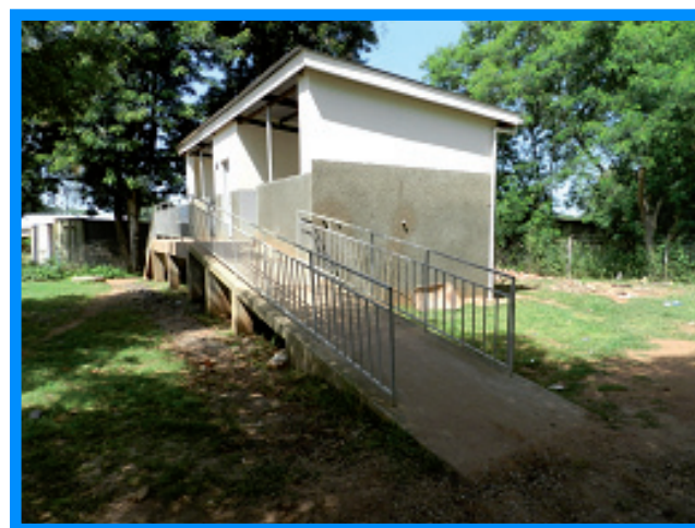
Public toilet by HORIZONT 3000 at St. Joseph Hospital Kitgum
