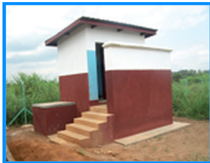
Public toilet with barrier (steep steps)
