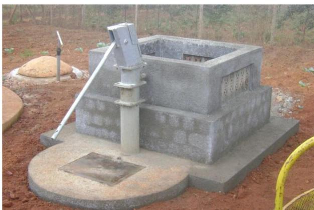
Silsoe design. Rainwater was then pumped into the tank and iron II sulphate at different doses was artificially introduced into the tank and the water pumped through the IRP to determine its efficacy. The study showed that up to 8 mg/l of water, the iron content was reduced to levels acceptable for drinking water by WHO. However for an initial iron content of 26 mg/l, the residual iron in the treated water was 5.93mg/l which is significantly higher than the WHO guideline.
