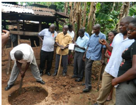
Step1: Laying ground for tank excavation
