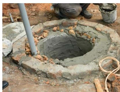
Step4: Fitting the pump holder
