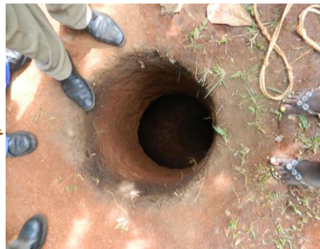
Step2: Complete excavation
