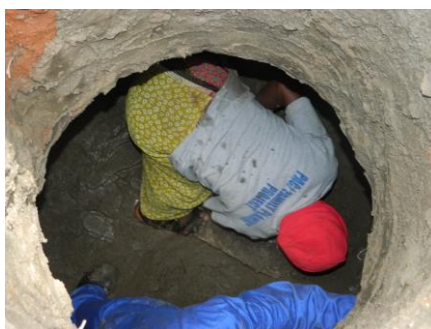
Step3: Plastering of the excavation
